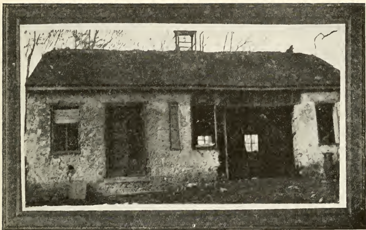
Old Academy Govanstown, Maryland
